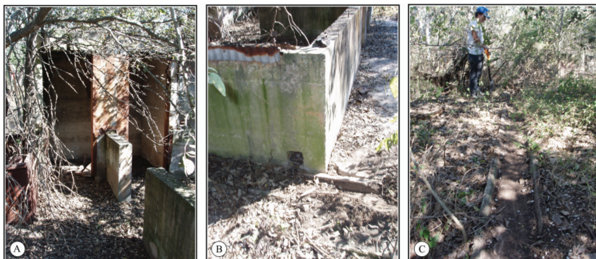
Figure 4-5. Details of concrete structure. Image A shows detail of rooms 3, 4, and 5 from the interior. Image B shows drainage hole from building. Image C shows drainage trough from building.
