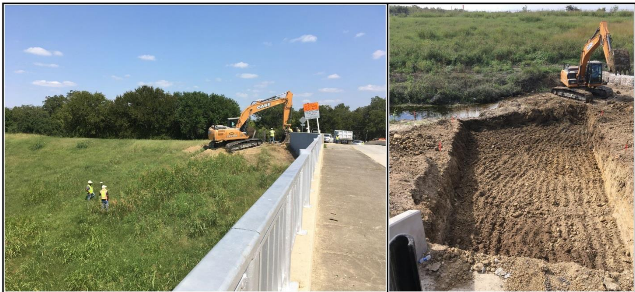
Figure 4-7. Beginning of the trench excavation for storm drain on Espada Road northwest of the Espada Acequia in Area 3 (left). The excavated storm drainage pipe outfall to Six-Mile Creek (right).
