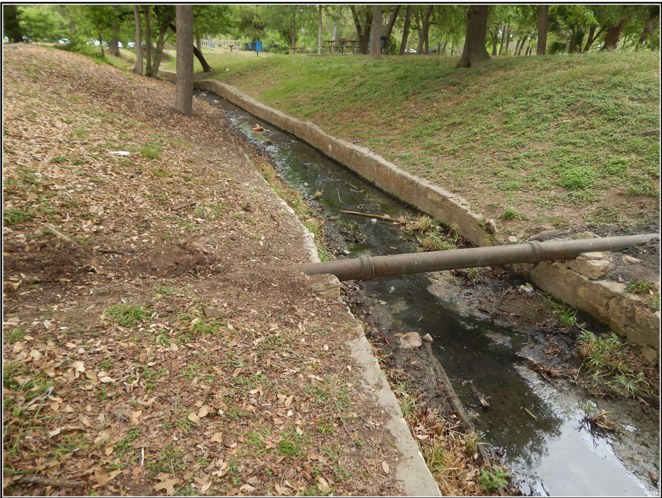
Figure 1-2. Southern margin of project area, facing east. Damaged sewer line laid directly across top of refurbished and fully exposed Upper Labor Acequia. The area excavated is to the left (north) side of this view.
