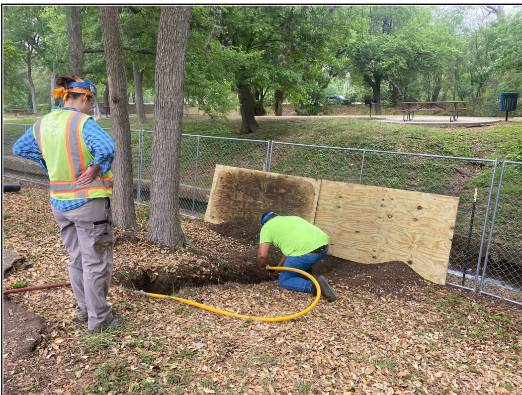
Figure 4-2. Air spade excavation and monitoring in progress (facing south).
