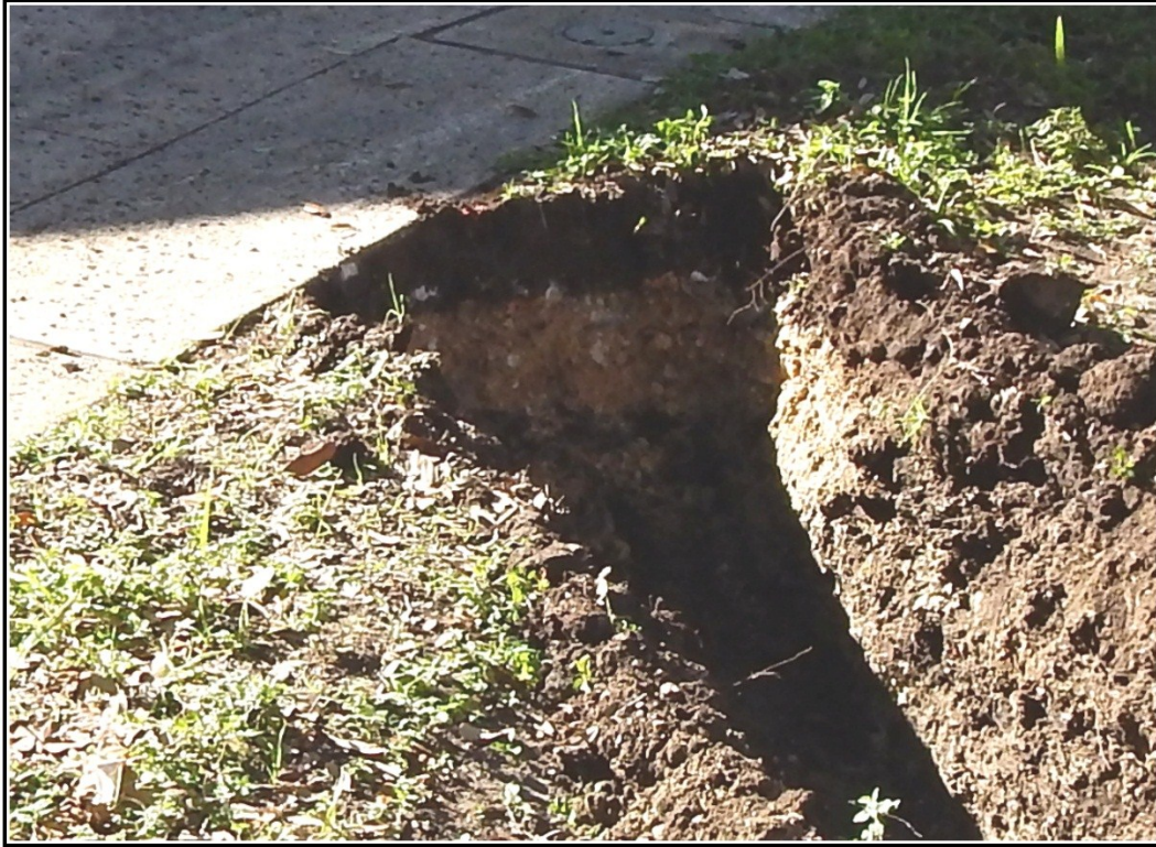
Figure 9. Trench excavated with boring bullet at water valve tie-in location, looking south. Note the disturbed sediment.
