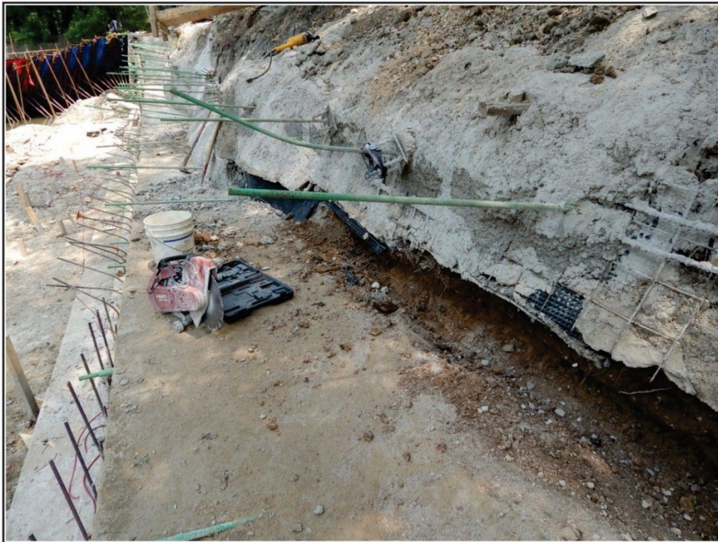
Figure 5-6. Excavations of French drain as documented May 10, 2016.
