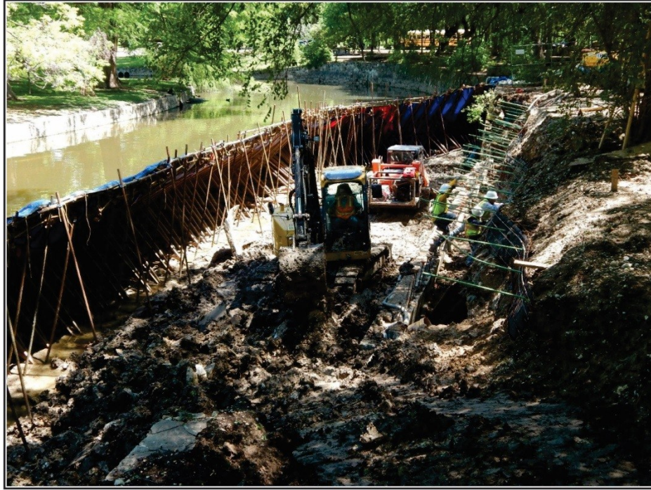
Figure 5-3. Dam installed to permit access to the riverbank.
