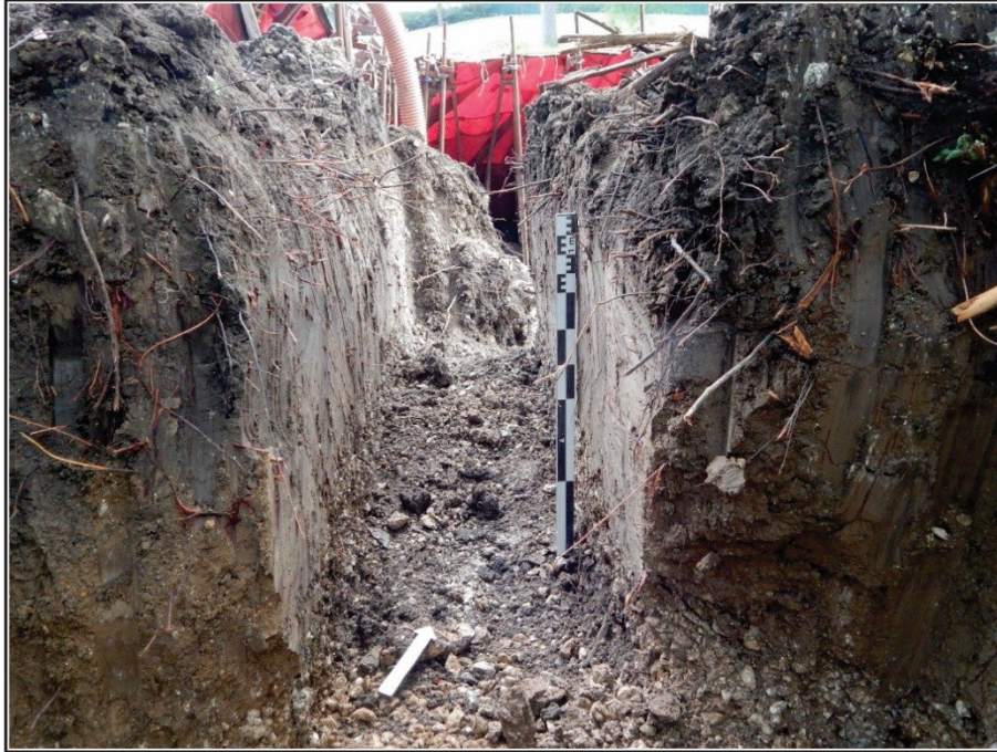
Figure 5-4. Drain pipe trench junction box excavation.
