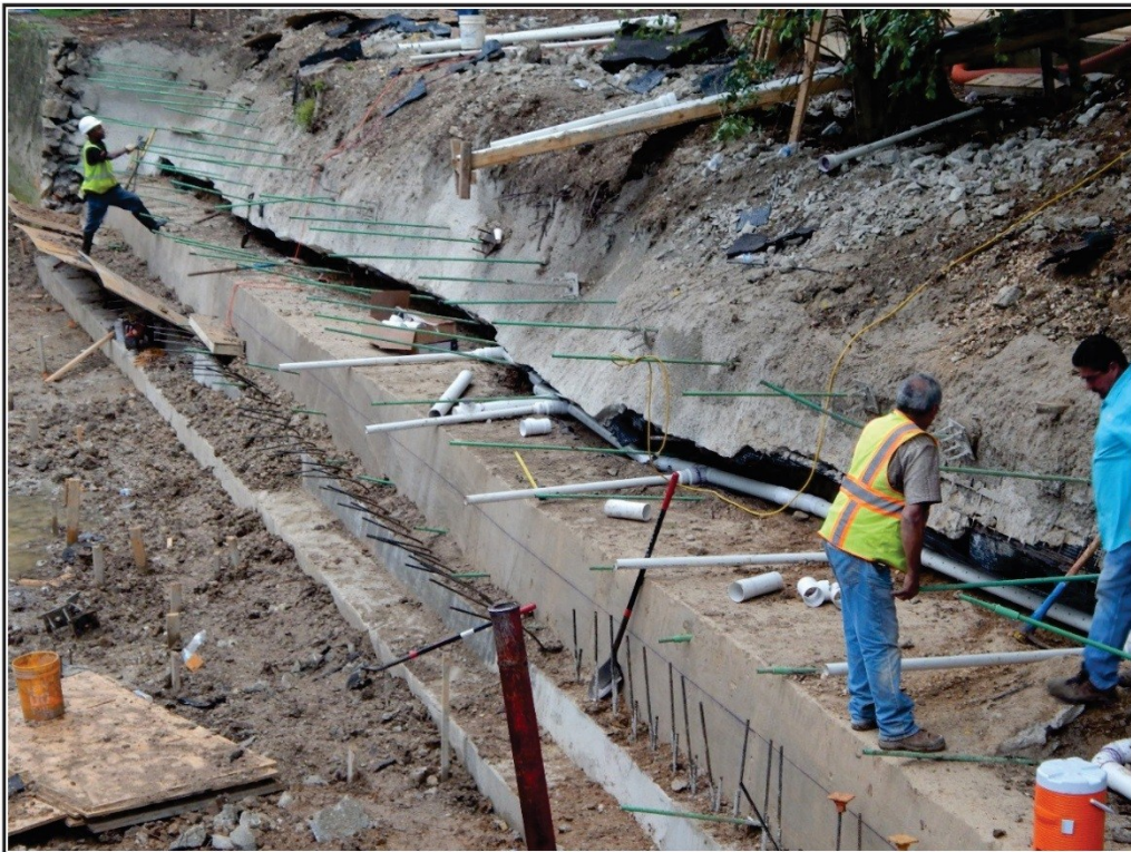
Figure 5-8. Installation of French drain.
