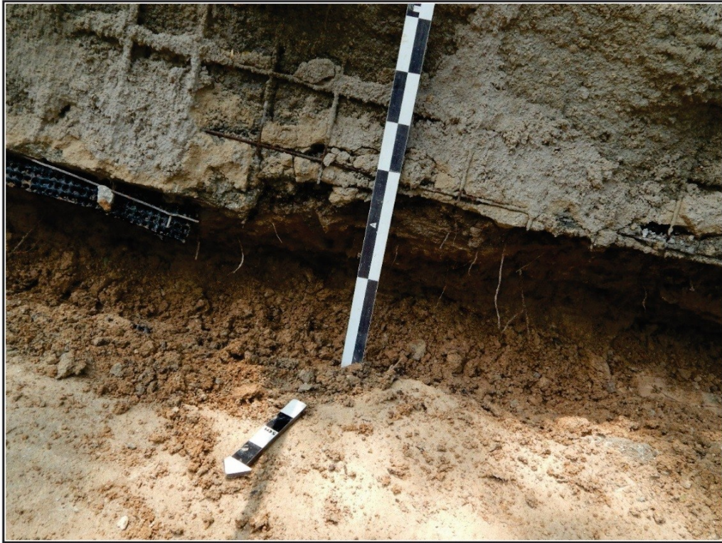
Figure 5-7. Vertical extent of excavation of French drain.
