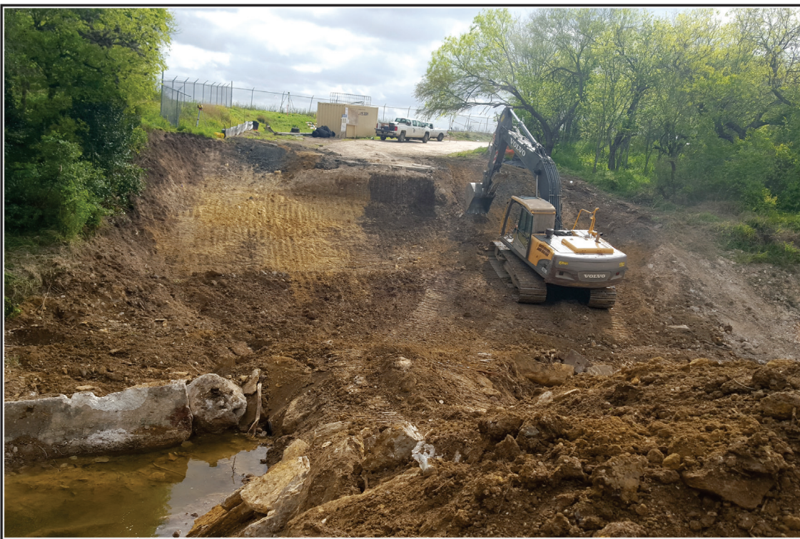
Figure 4-2. Grading of east bank of the creek for riprap.
