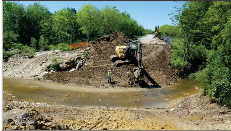
Figure 4-9. Grading of slope on east bank of Sixmile Creek.
