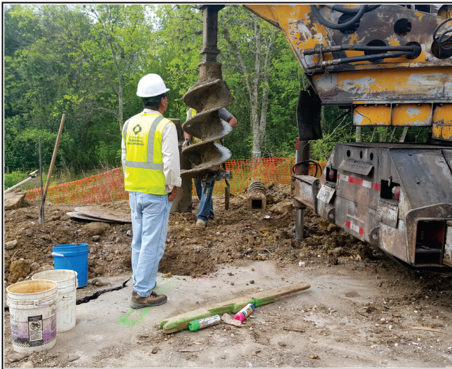
Figure 4-4. Drilling of holes for pier installation on the west bank.
