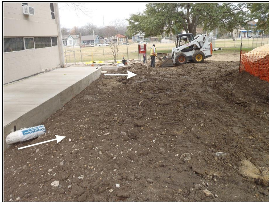
Figure 4-6. New sidewalk against north wall of Playhouse. Note drainage pipes extending from sidewalk.
