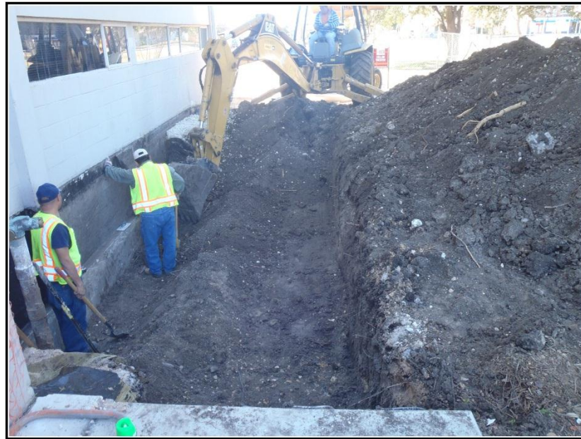
Figure 4-3. Trench 1 being excavated by backhoe and shovels.
