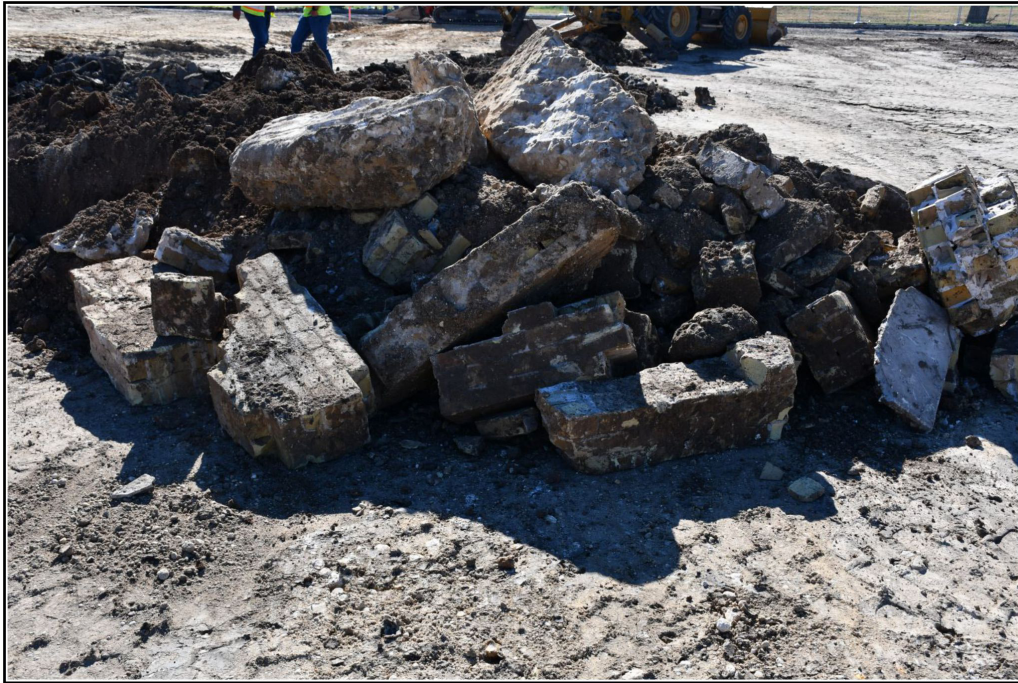
Figure 5-9. Material removed during demolition of brick structure. Note large chunks of concrete, brick sitting in concrete.
