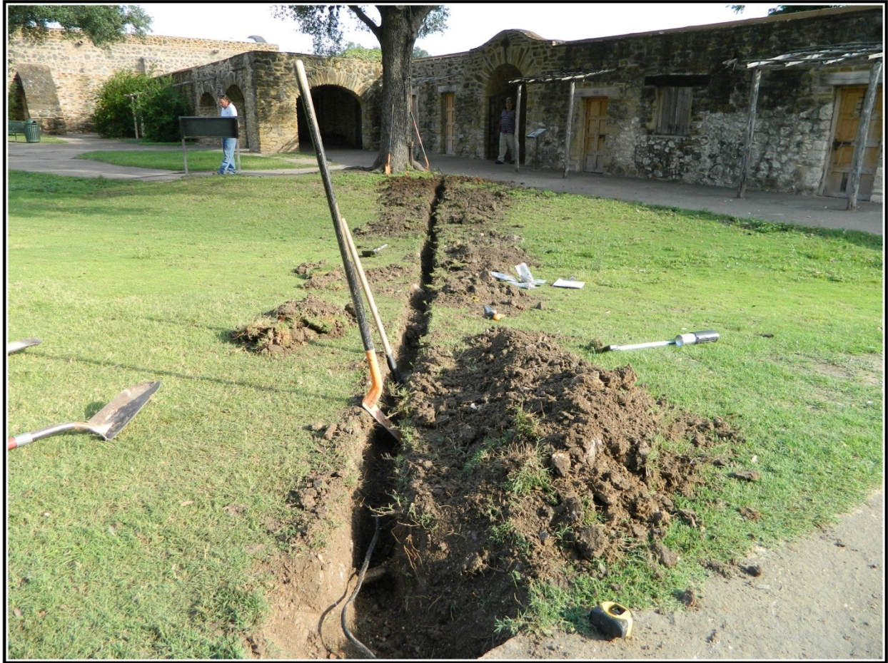
Figure 4-7. Trench 2 running from in front of the church to a junction box next to the tree.
