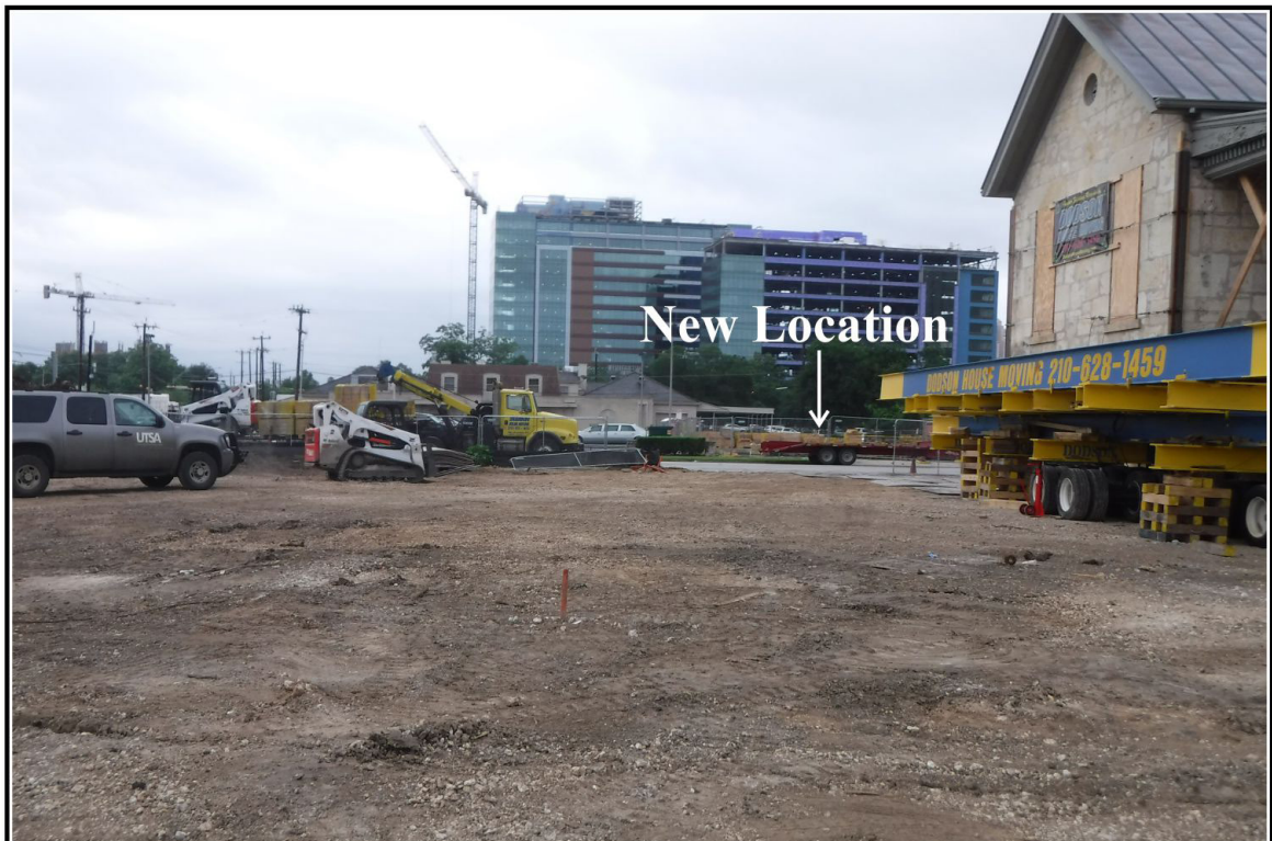
Figure 4-9. View of the house after being turned 180 degrees in preparation for move across the street (view east).
