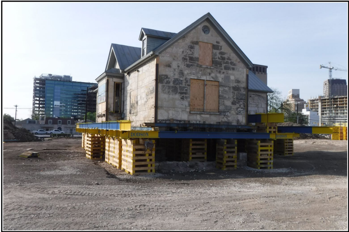
Figure 4-8. View of house raised above original footings.
