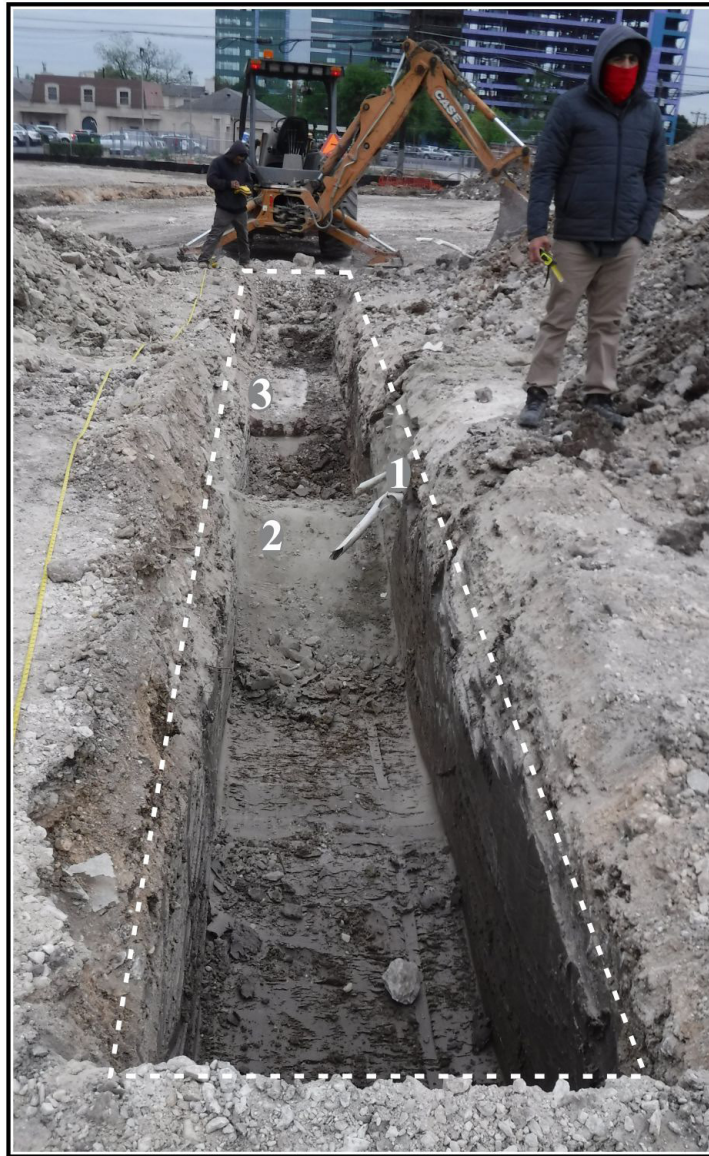
Figure 4-4. Backhoe Trench 1, excavation complete (view east): 1) irrigation lines, PVC; 2) concrete berm, possible duct bank; and 3) concrete pad.
