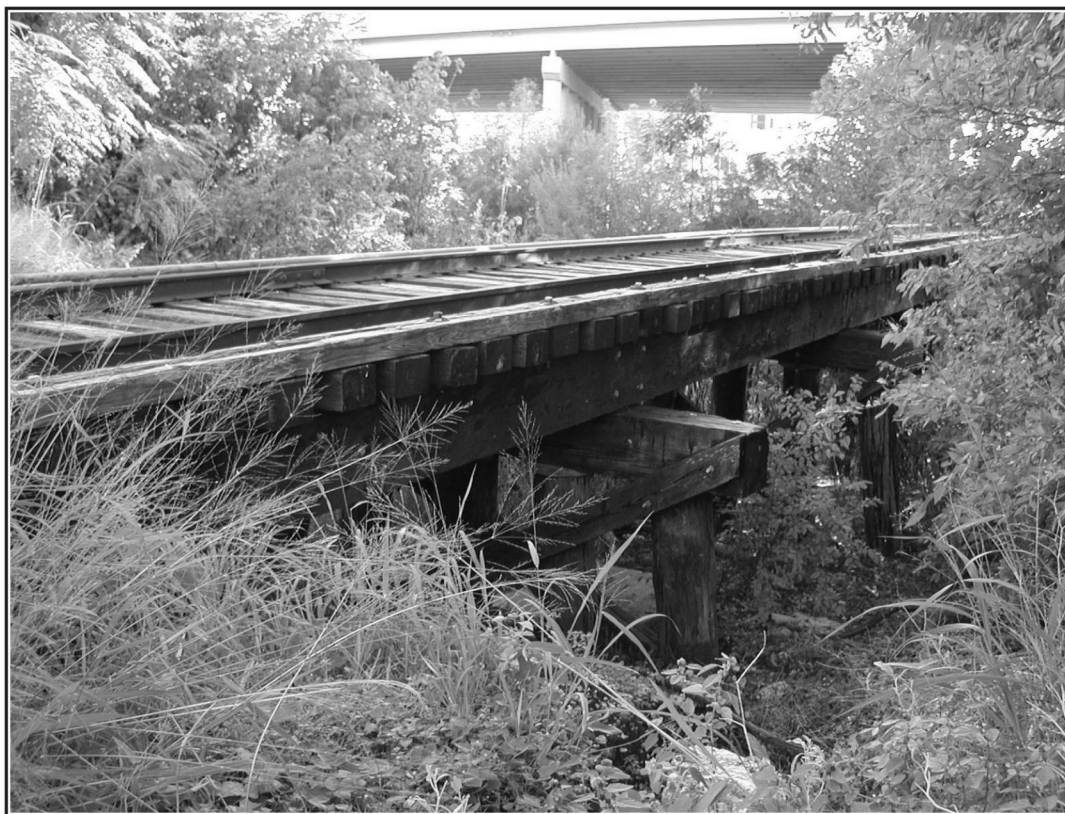
Figure 2-8. Wooden trestle bridge located between Camden Street and IH-35.
