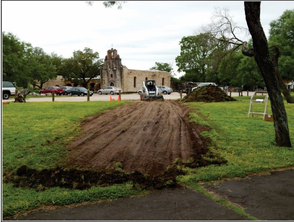
Figure 4-4. Completed swale with sloped edges.
