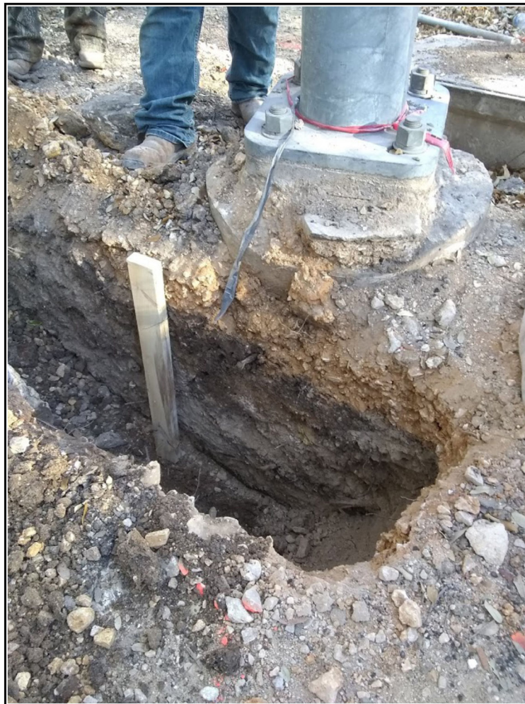
Figure 4-4. Trench excavation for the CPS electrical lines at corner of W. Travis Street and N. Flores Street. Note light pole and associated electrical box at upper right indicating disturbances in this portion of the trench (facing northwest).
