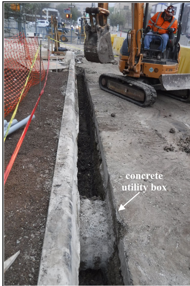
Figure 4-5. CPS electrical line excavations along the western end of W. Travis Street. Note the concrete utility box at the bottom of the picture indicating disturbances in this portion of the trench (facing west).
