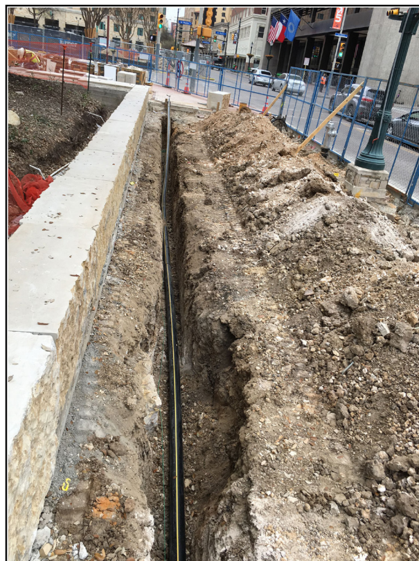
Figure 4-3. The eastern end of the CPS gas line trench with line installed.
