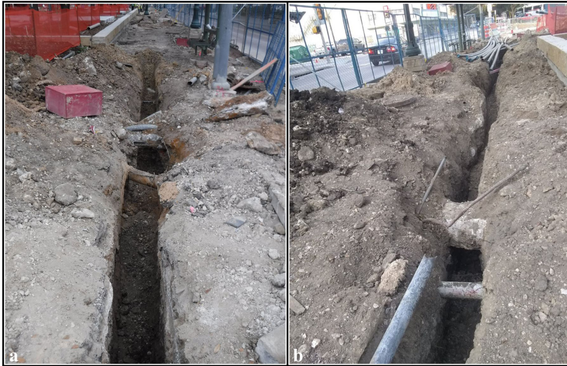
Figure 4-2. Excavation for the CPS gas line encountered: a) existing utility lines (facing east) and b) existing utility lines and concrete easements (facing west).
