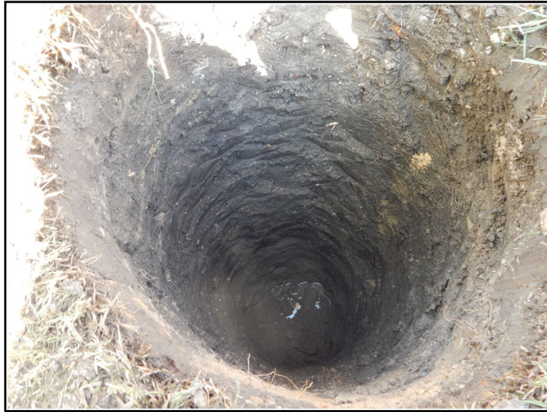
Figure 4-3. Pole hole excavated in Jesus Alley. Note sand fill in west wall.
