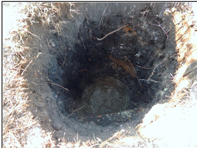
Figure 4-4. Pole hole excavated at 1619 Monterey; note copper pipe and utility trench fill.
