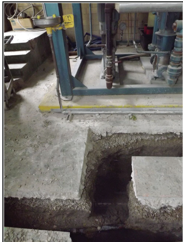
Figure 4-35. An example of trenching to repair pipes in the Boiler Room.
