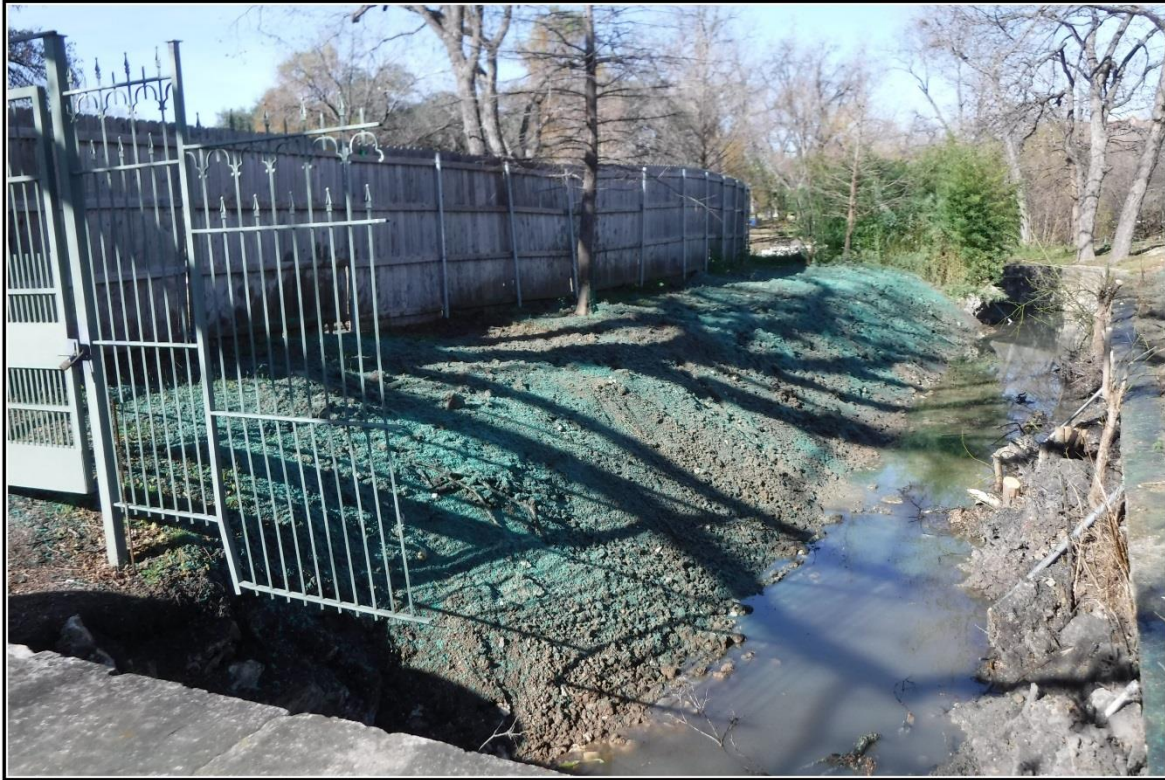
Figure 4-8. Canal banks treated with grass seed and fertilizer.
