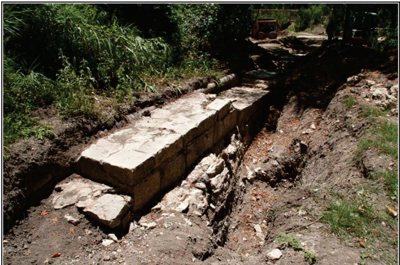
Figure 5-16. Northern terminus, west face. Nineteenth-century ashlars superimposed on eighteenth-century Spanish Colonial dam.
