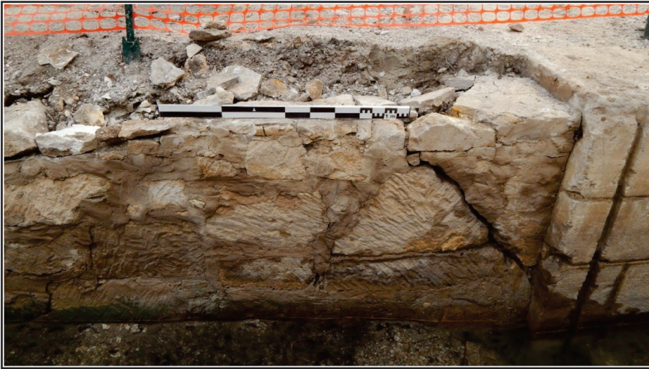
Figure 5-10. Upper channel wall (east) showing mixed construction and visible damage.
