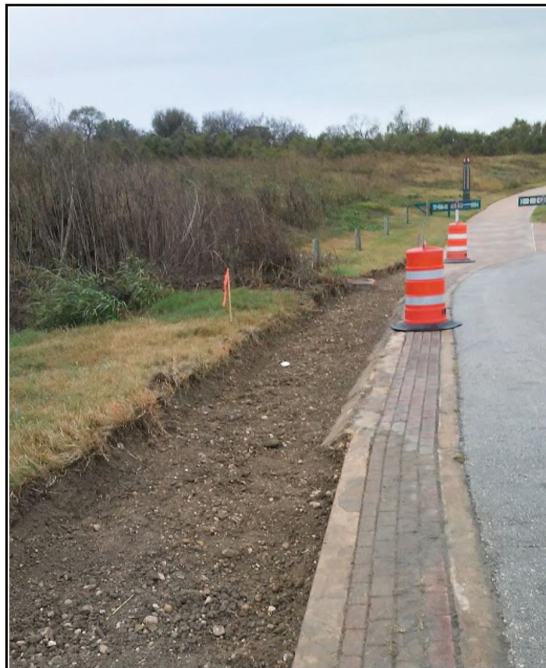
Figure 4-9. Excavations on Camino Coahuilteca for sidewalk installment, with existing sidewalks to the north.
