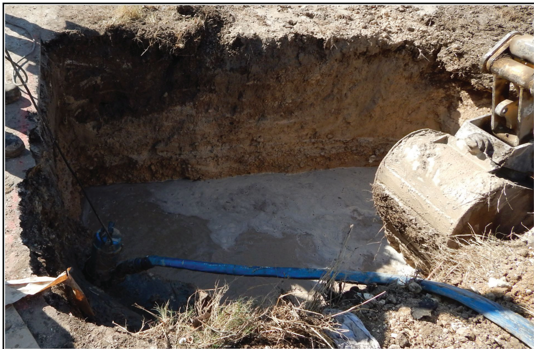
Figure 4-7. Flooded footing trench for pedestrian bridge crossing the San Juan Acequia. The layered appearance in the lighter portion of the soil profile is an artifact of the trench being repeatedly flooded and pumped during excavation. The profile did not exhibit this layering during the initial excavation.
