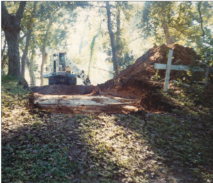
Figure 5-4. Photograph of Gradall scraping in progress.
