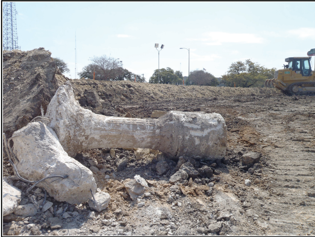
Figure 5-5. Foundation piers from the former K-Mart complex that occupied the tract.
