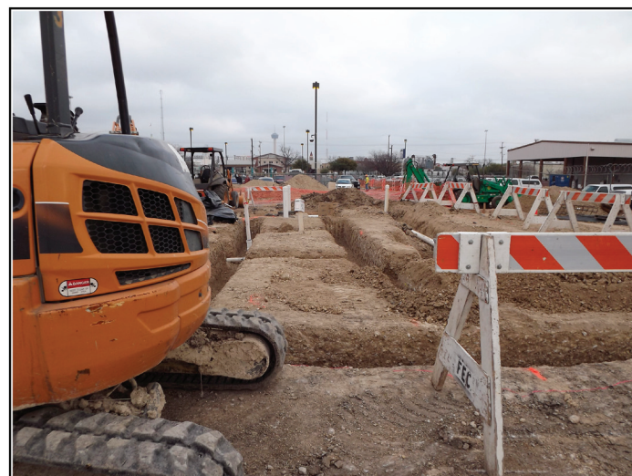
Figure 4-8. Trenches excavated into fill introduced to achieve the required grade in eastern half of APE.
