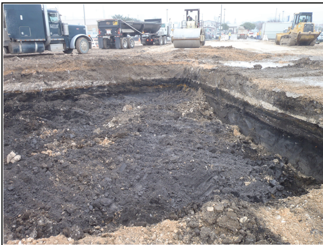
Figure 4-5. Partially excavated gasoline storage tank pit.
