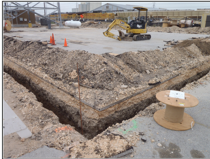
Figure 4-7. Trenches excavated to receive pipes leading to the gasoline pumps from the storage tanks.
