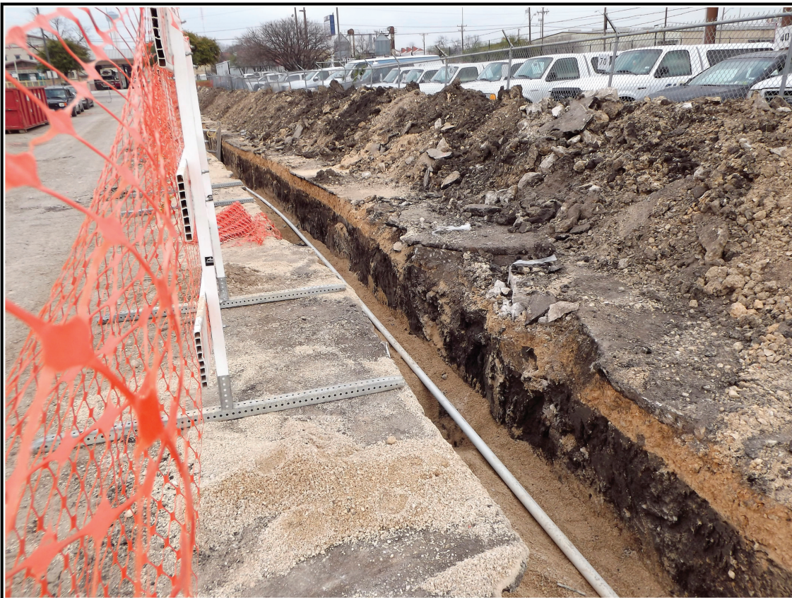
Figure 4-10. Trench with installed electrical conduit leading from the gasoline pumps toward Frio Street.
