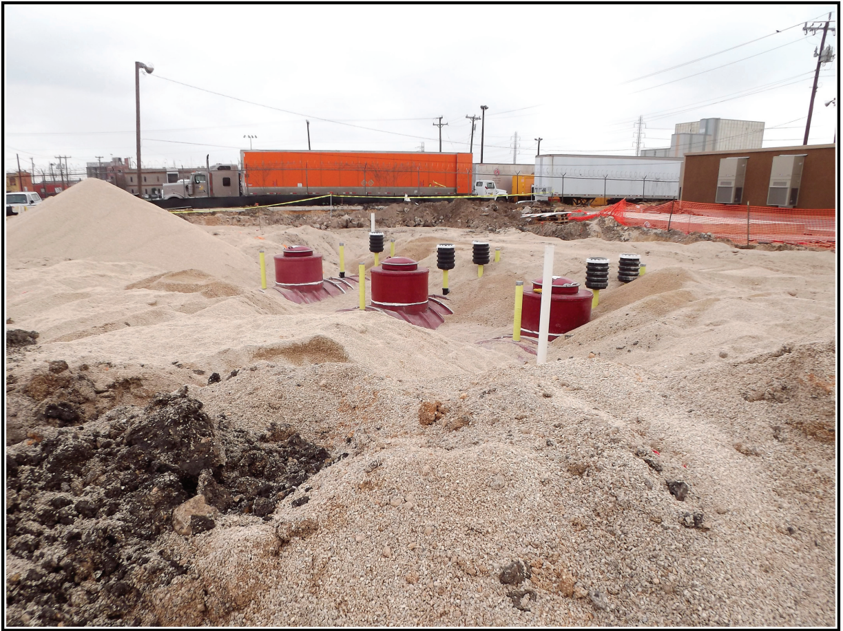
Figure 4-11. Gasoline storage tank pit being filled with crushed limestone.
