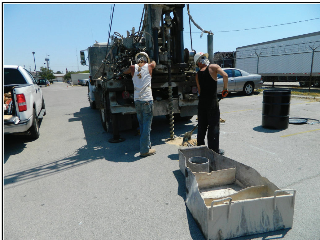
Figure 4-1. Geotechnical coring in progress at the fueling station facility.
