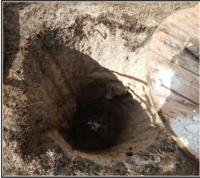
Figure 4-5. Hydro vacuumed pole excavation.
