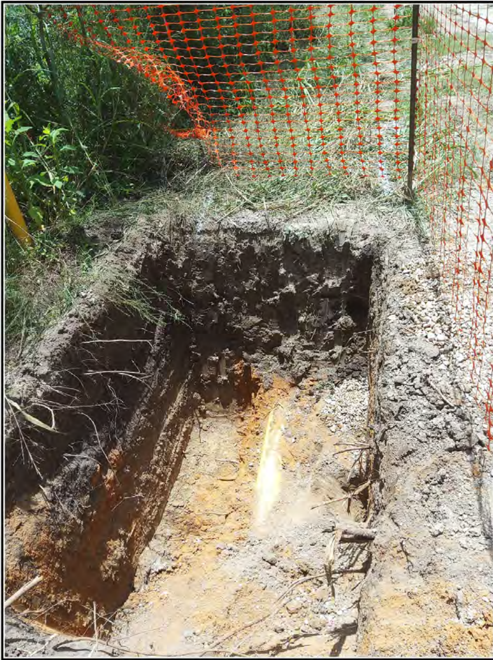
Figure 5-12. Gas line excavation within project area.
