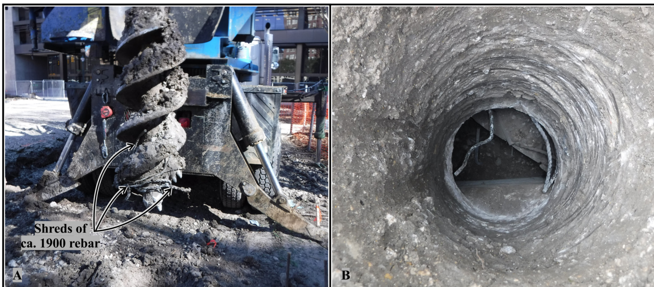
Figure 4-5. A. Auger at Pier 12—note shreds of rebar on auger; B. Looking down into the 18-inch diameter hole—broke through rebar-reinforced concrete.
