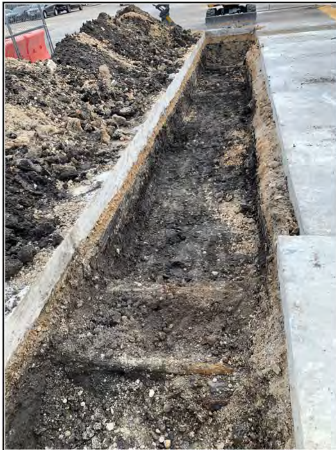
Figure 4-3. Trench with shallowly buried utilities.
