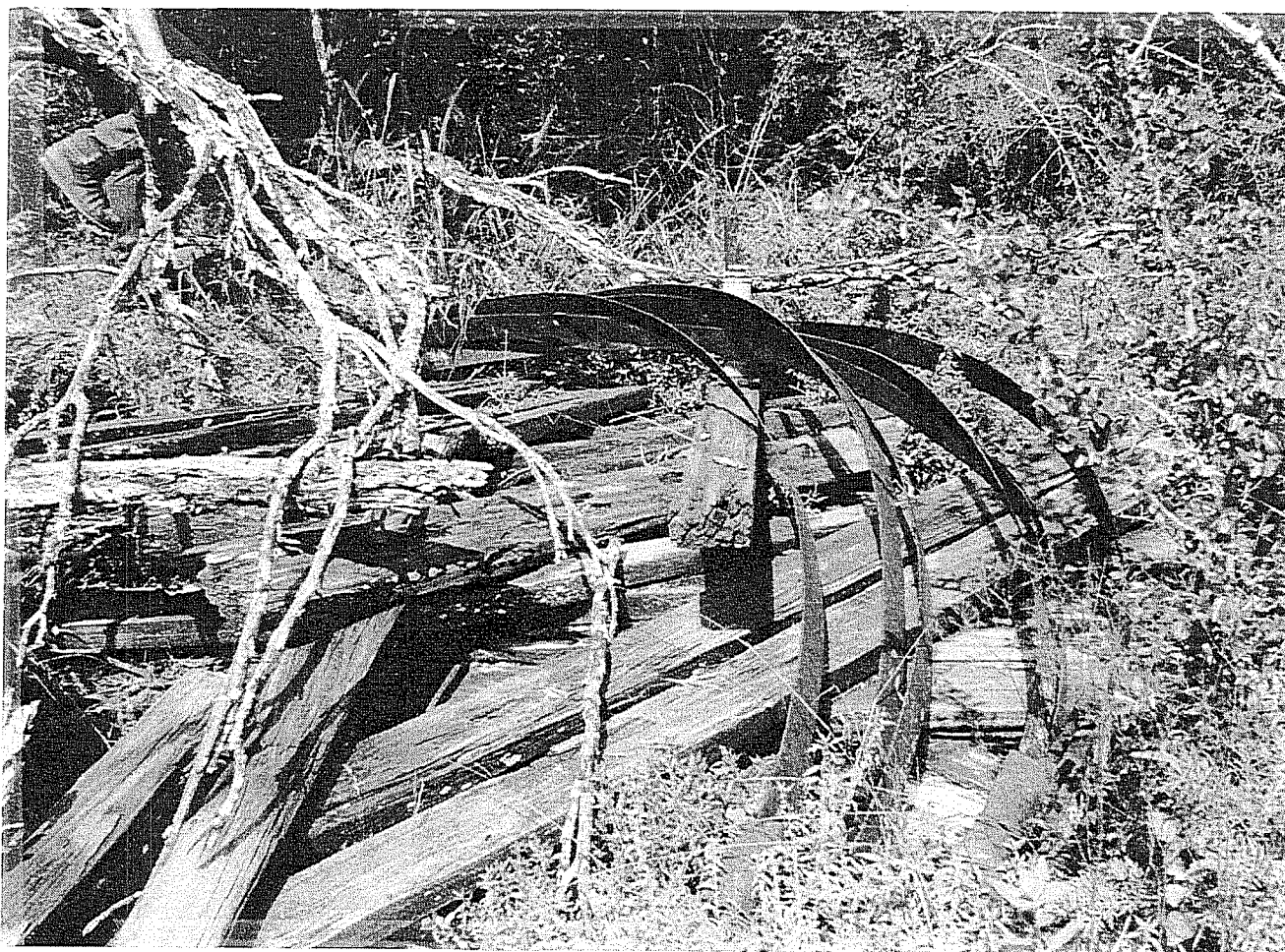
Figure 13-9. Collapsed cypress water tower at 41BX1128.
