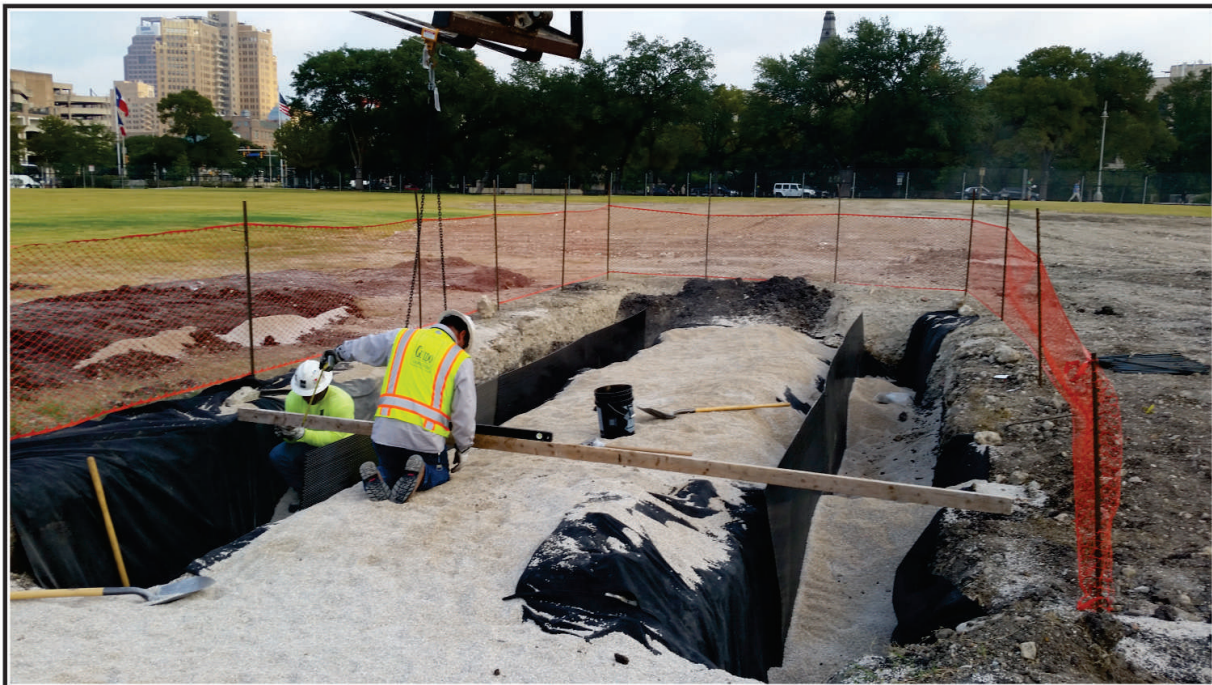
Figure 4-12. Guido Brother's crew measuring distance between outer wall steel plates on northern end, facing north.
