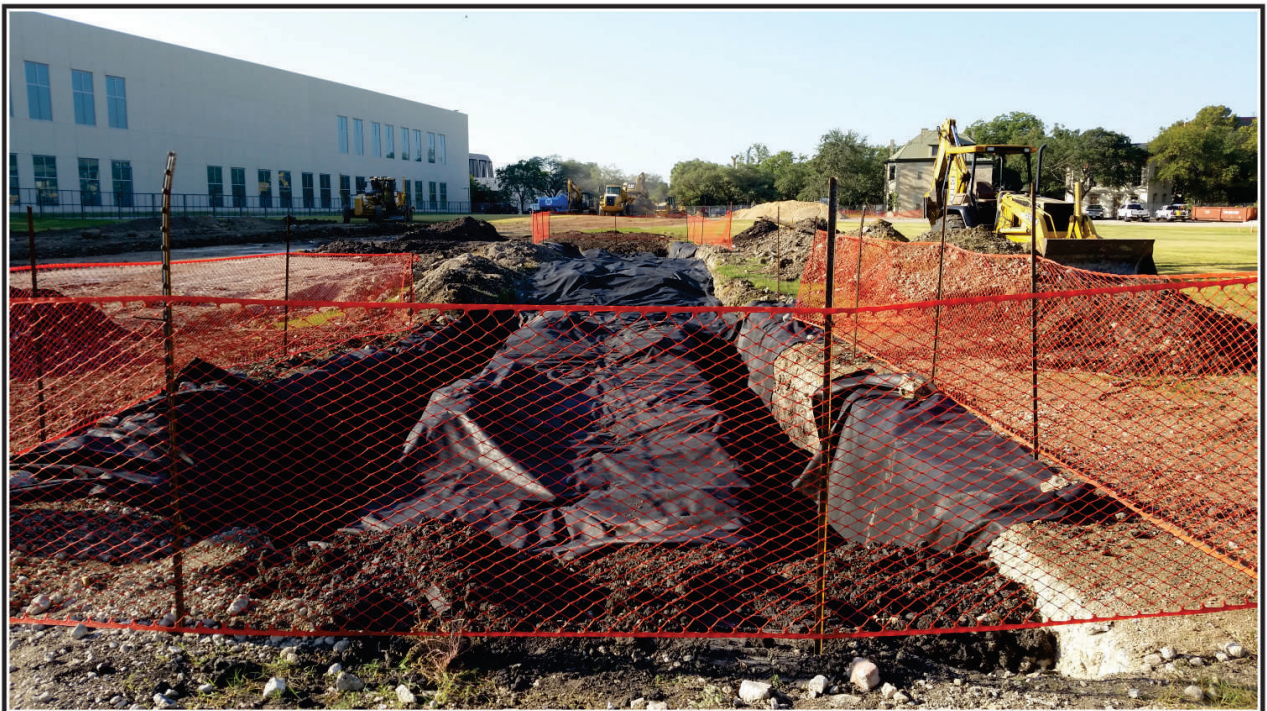
Figure 4-10. Black felt landscape fabric covering the acequia, facing south.
