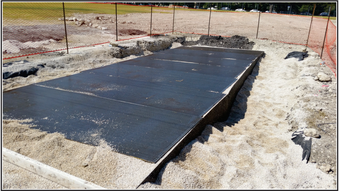
Figure 4-13. Northern end encased with gravel and three sides of plates, facing northwest.
