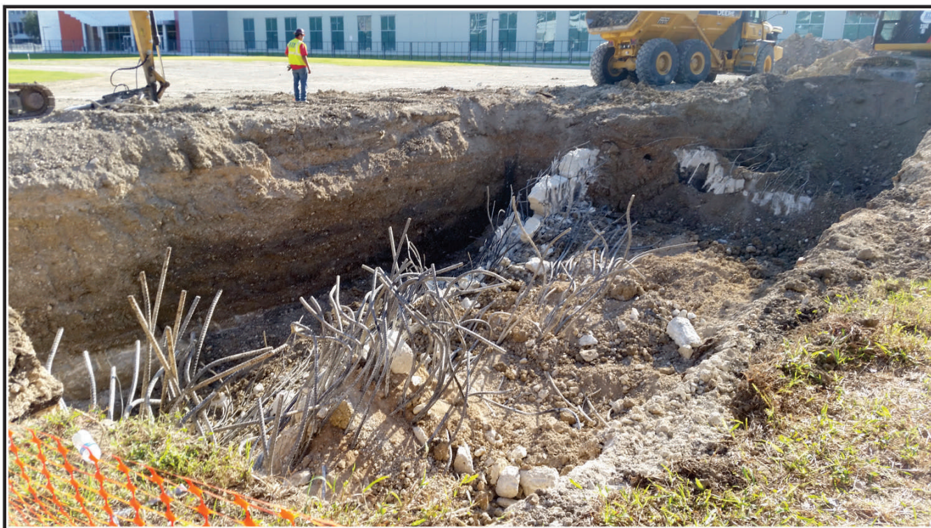
Figure 4-3. Vault excavation, note concrete and rebar.
