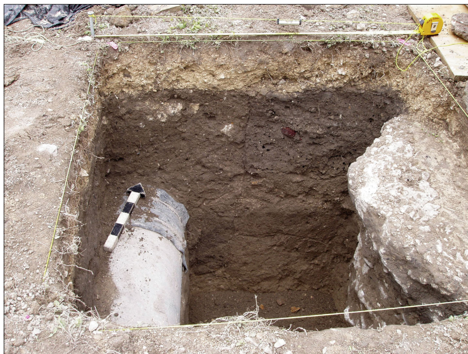
Figure 3-11. Pipe and buttress exposed in Unit F.
