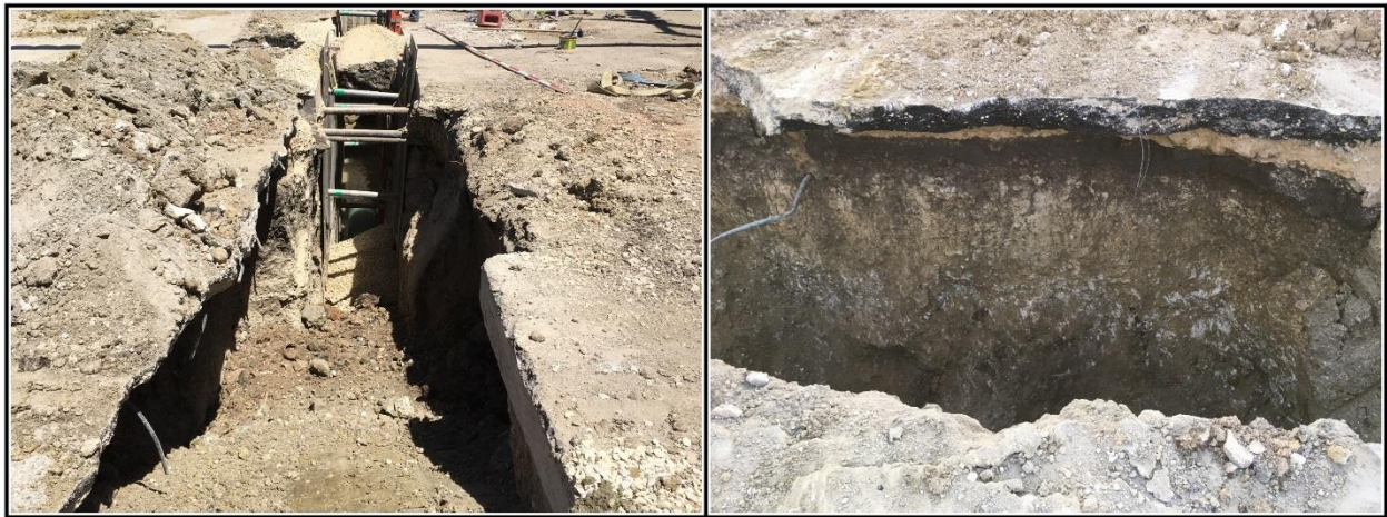
Figure 4-3. Excavation for sewer line showing evidence of previous construction (left). Image on the right shows a similar soil, clay with caliche, as observed during the manhole excavation.
