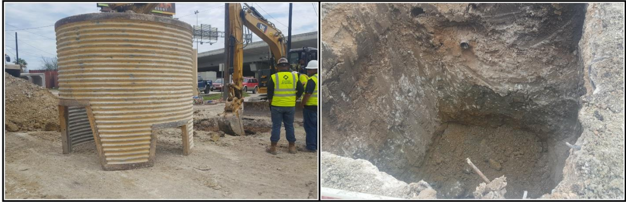
Figure 4-2. Excavation for manhole (left). Soil profile of excavation showing clay with caliche (right).
