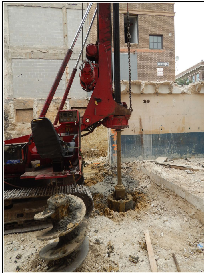
Figure 5-2. Location of pier hole starting surface; note that it is below the original ground surface.
