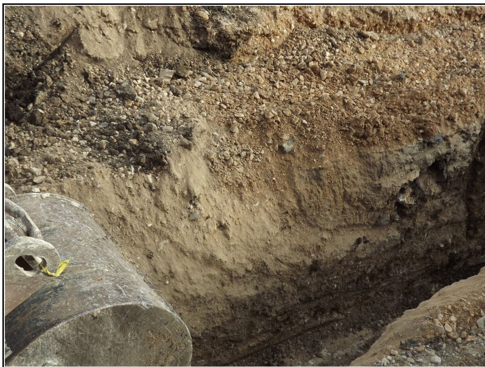
Figure 5-8. Utility trench profile, note a top zone of construction fill over clay.
