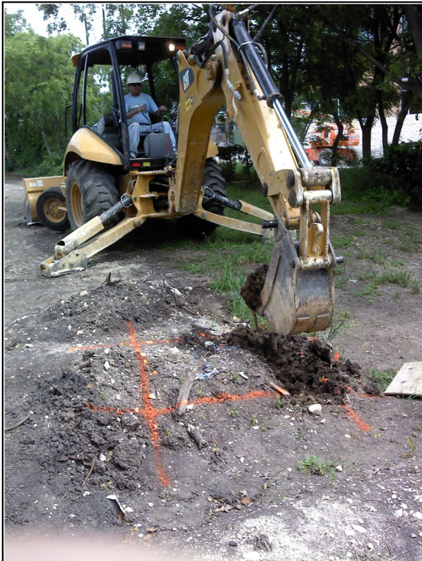
Figure 7-2. Backhoe excavating trenches for the installation of light posts along the hike and bike trail.
