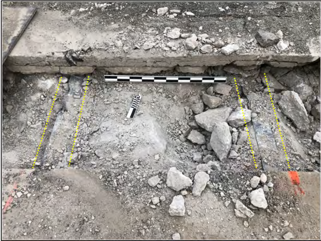
Figure 4-4. Narrow exposure of track remnants prior to tie removal.
