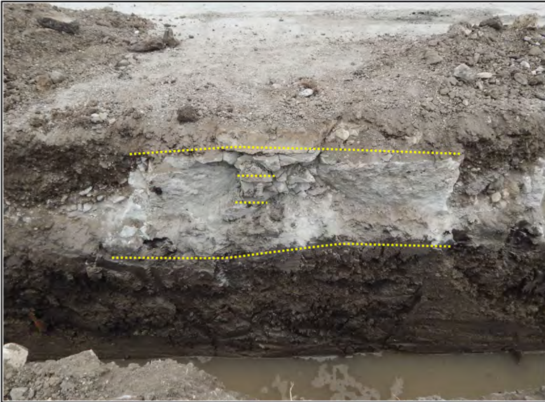
Figure 4-2. Example track profile with concrete and I-rail tie exposed; note lack of gravel foundation layer.
